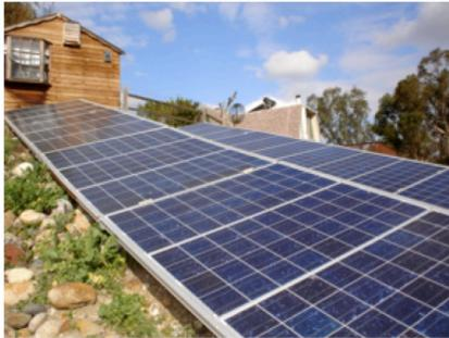
Multicrystalline 2.8 kW, ground-mounted.
